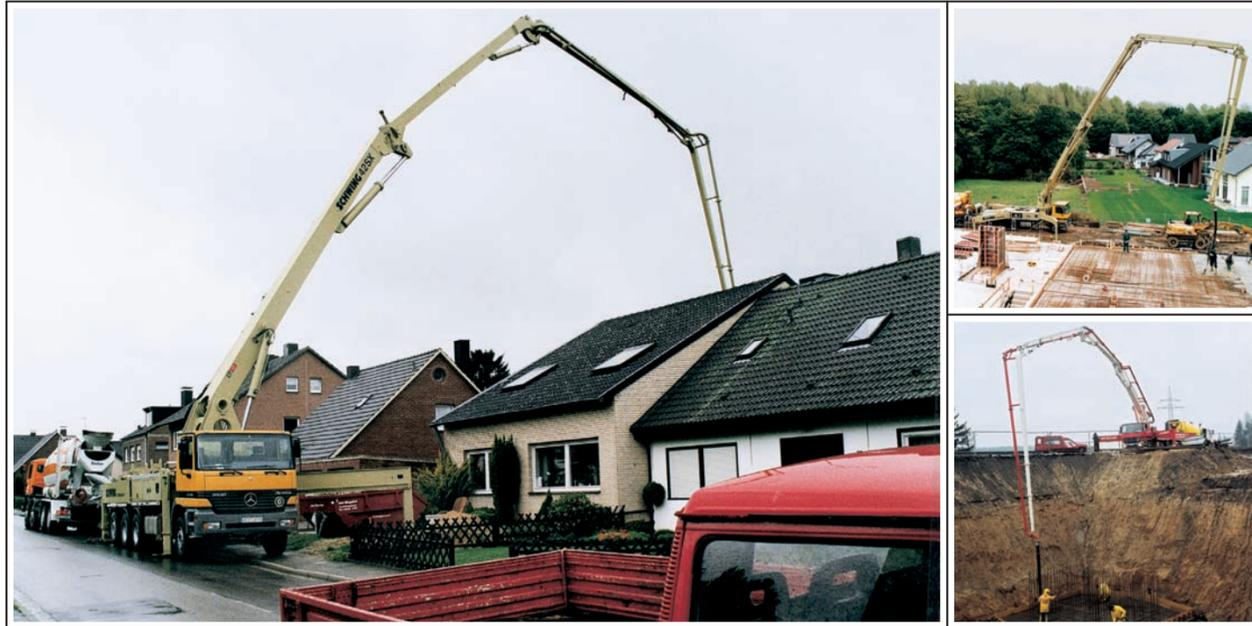
SCHWING **EASy** – our optional single-sided set-up for fail-safe operation when the pump can only be stabilized on one side. An absolute must for machines that need
